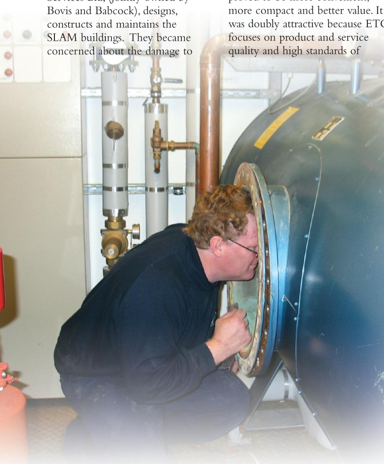
Inspection of the calorifier's heat exchanger
